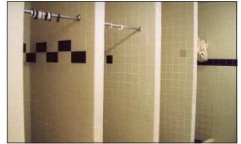
Finished shower stalls.
