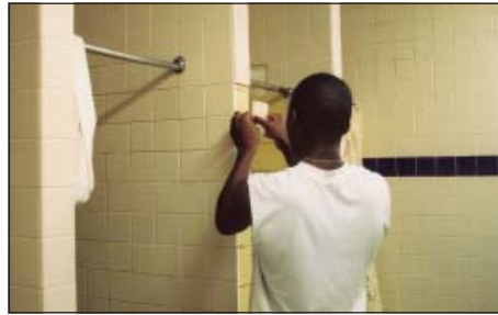
Replacing old tile.
